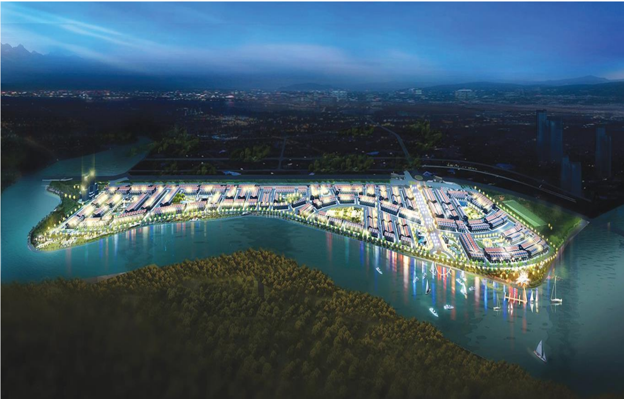
Bac Ha Thanh Residential Area in combination with urban gentrification in Binh Dinh
