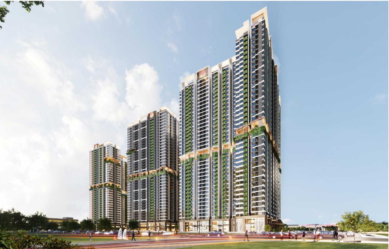
Thuan An 1 & 2 High-rise Residential complex in Binh Duong
